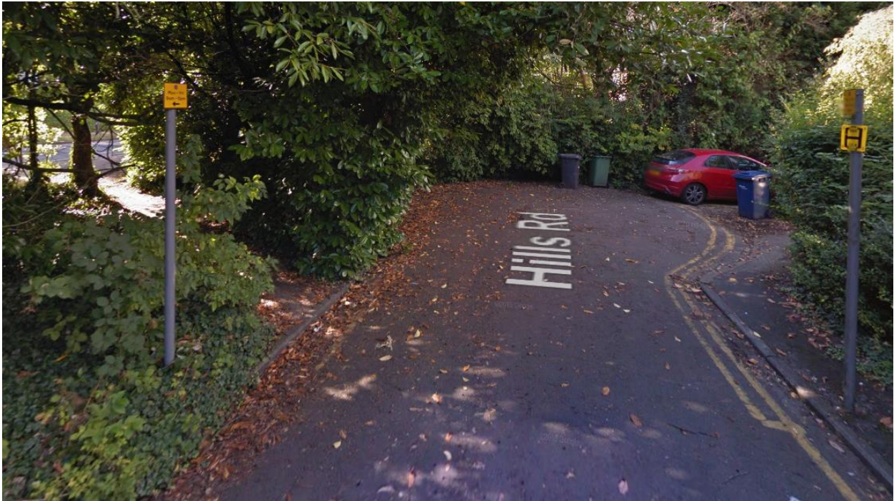
Figure 5: Existing informal footway between Hills Rd and parallel residential access road
