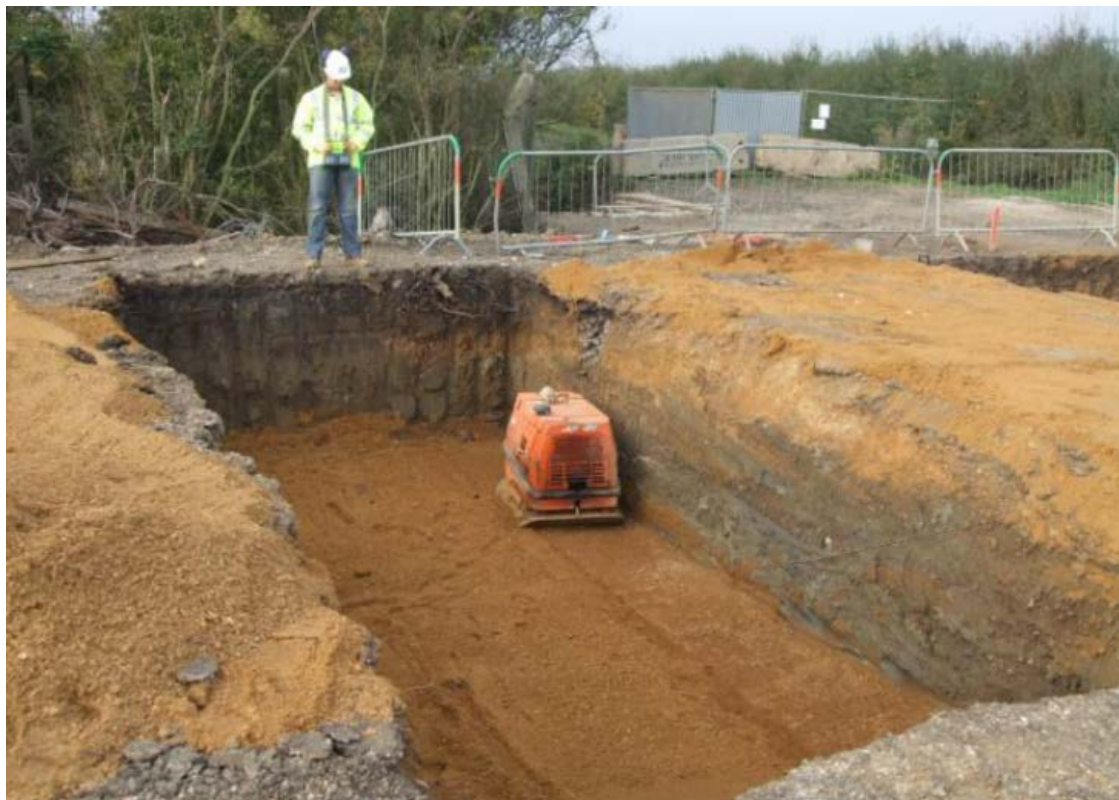
Figure 2: Shallow foundation [2-Fig 7]. 821 of these are to be re-excavated, deepened and re-instated
