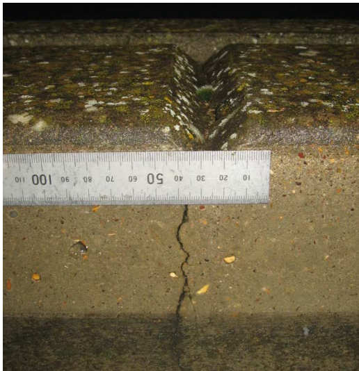
Figure 5: Crack originating at V-notch. Measured photogrammetrically as 0.6mm.
