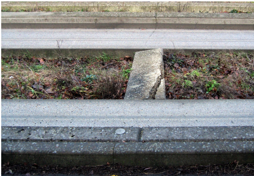
Fig 7 Fractured centre spacer. The spacer has pitched forward. The top of the beams have apparently rolled inward and pinched the spacer, as indicated in Fig 2c, above, resulting in fractures at both ends.
